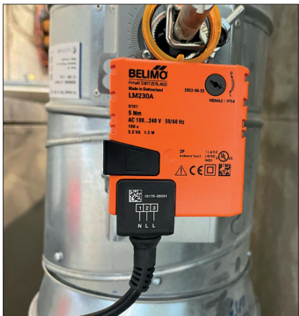
Obr. 5. Servopohon Belimo LM230A
